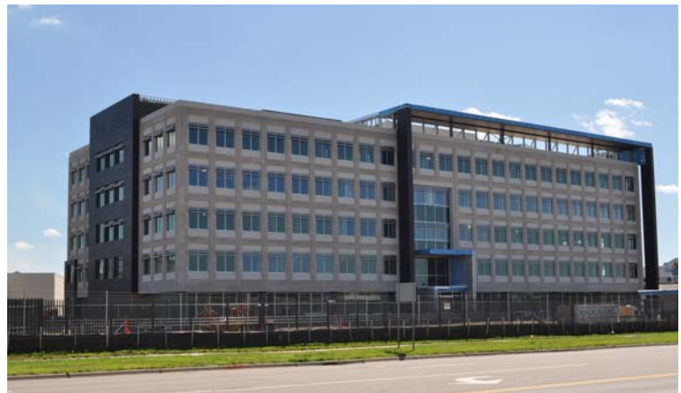
FBI Field Office, Brooklyn Center. Photo by Metropolitan Council.
